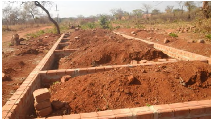
Foundation for two married student houses
